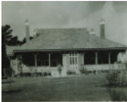
B2153 Mine Manager's Residence
