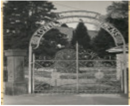
B2691 Cast iron fence and gateway
