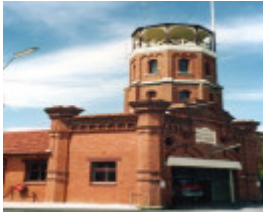
B4924 Ballarat East Fire Station Tower
