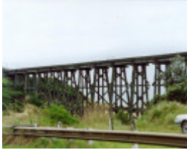
B2949 Trestle Bridge Kilcunda
