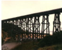
B2949 Kilcunda Bridge
