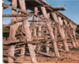
B2949 Kilcunda Bridge
