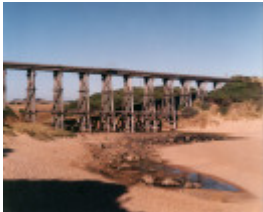
B2949 Kilcunda Bridge
