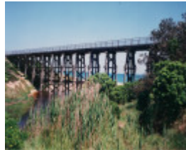
B2949 Kilcunda Bridge
