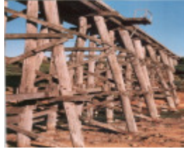
B2949 Kilcunda Bridge
