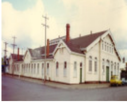
B5305 Drill Hall
