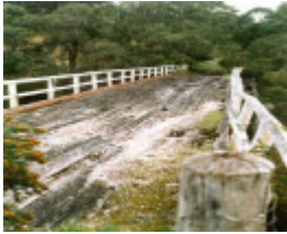
B6923 Springdallah Bridge
