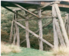
B6923 Springdallah Bridge
