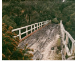
B6923 Springdallah Bridge
