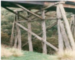
B6923 Springdallah Bridge
