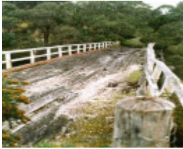
B6923 Springdallah Bridge
