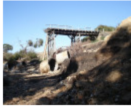
B6923 Springdallah Bridge remnants
