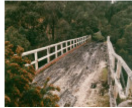
B6923 Springdallah Bridge
