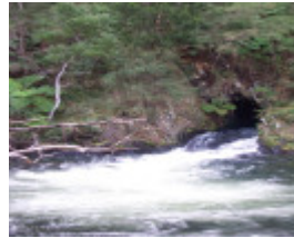
B7176 Thomson River Diversion Tunnel
