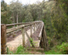
B1525 Noojee Rail Trestle Bridge
