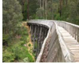
B1525 Noojee Rail trestle Bridge
