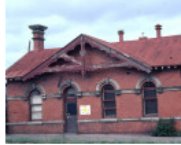
B0276 Ballarat Railway Station
