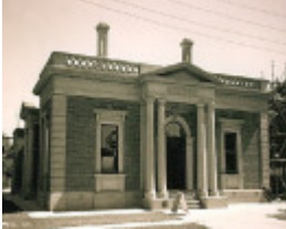
B2009 Former Shire Hall
