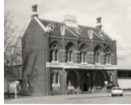
B2655 Old Shire Hall
