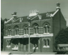
B2655 Old Shire Hall
