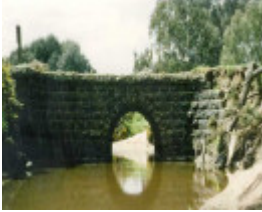
B5283 Bluestone Bridge
