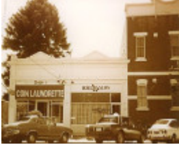
B6234 Former Holmfield's Site
