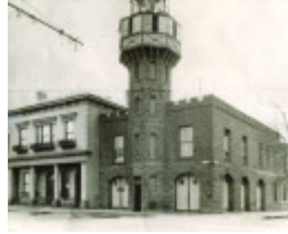
B3282 Former Ballarat Fire Station
