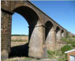
MALMSBURY RAIL BRIDGE SOHE 2008
