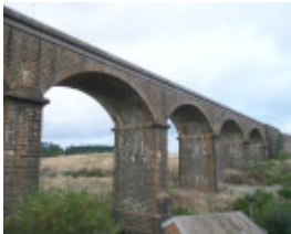
MALMSBURY RAIL BRIDGE SOHE 2008
