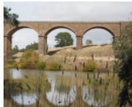
MALMSBURY RAIL BRIDGE 2020
