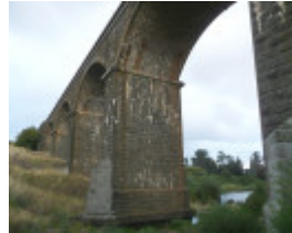
MALMSBURY RAIL BRIDGE SOHE 2008
