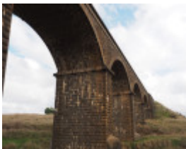
MALMSBURY RAIL BRIDGE 2020
