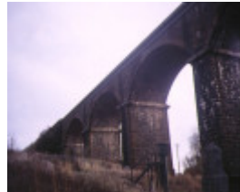
1 rail bridge over coliban river malmsbury side elevation apr1995
