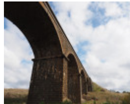
MALMSBURY RAIL BRIDGE 2020
