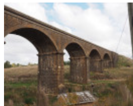
MALMSBURY RAIL BRIDGE 2020
