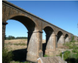
MALMSBURY RAIL BRIDGE SOHE 2008
