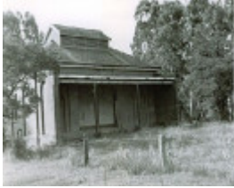
B1311 Pumping station
