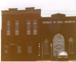
B4178 Former Shackell's Bond Store
