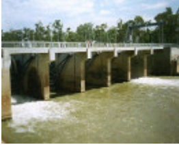
B6516 Torrumbarry Weir
