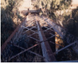
B7055 Glenmona Bridge
