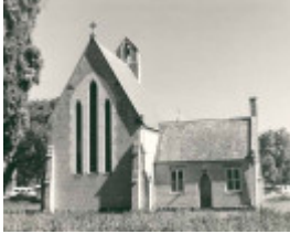
B3355 St Paul's Church Front View
