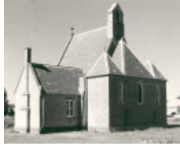
B3355 St Paul's Church Back View
