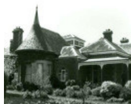
B1709 Coragulac House South Side
