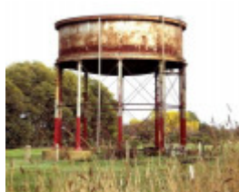
B4458 Railway Station Watertower
