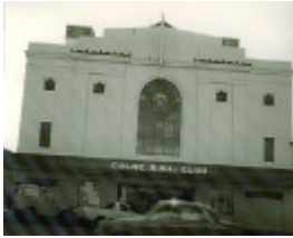
B5116 RSL Building
