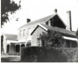
B1401 Timboon House - Old Geelong Rd, Timboon
