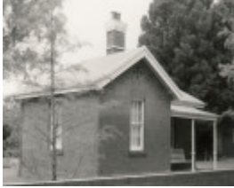
B2201 Former Survey Office
