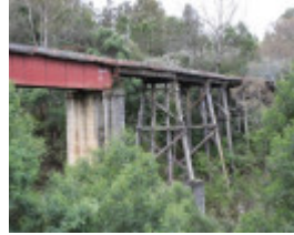
B6943 Boggy Creek Bridge
