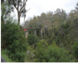
B6943 Boggy Creek Bridge
