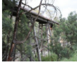
B6943 Boggy Creek Bridge Piers
