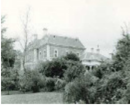
B1450 Golf Hill homestead Complex, Shelford
