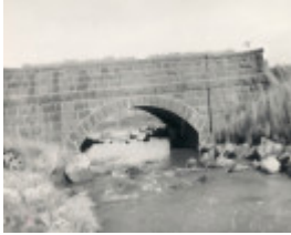
B1503 Road Bridge Rodewood
