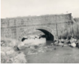
B1503 Road Bridge Rodewood
