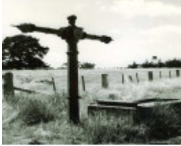
B2358 Stand Pipe & Trough
