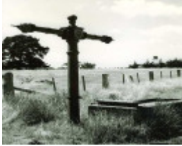
B2358 Stand Pipe & Trough
