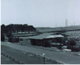
B6788 Former Railway Goods Shed
