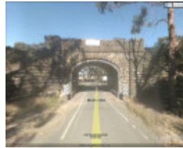
B2551 Bluestone Bridge
