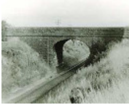
B2587 Road Bridge
