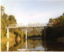
B2260 Genoa River Bridge
