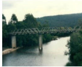
B2260 Genoa River Bridge
