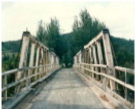
B2260 Genoa River Bridge
