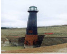
B7048 Outlet Tower
