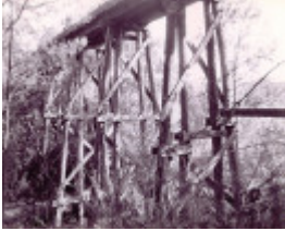
B6947 Hospital Creek No1 Bridge
