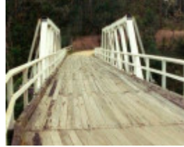
B6847 Murrindal Bridge
