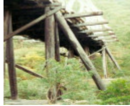
B6847 Murrindal Bridge
