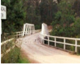
B6847 Murrindal Bridge
