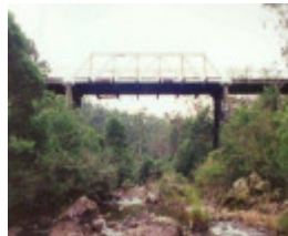
B6847 Murrindal Bridge
