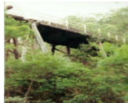
B6847 Murrindal Bridge
