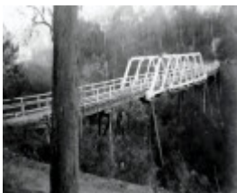
B6847 Murrindal Bridge
