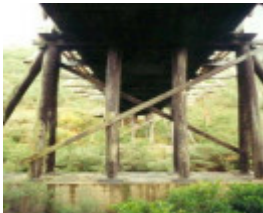
B6847 Murrindal Bridge
