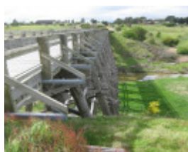
B7086 Nimons Bridge deck 2011
