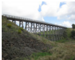
B7086 Nimons Bridge 2011
