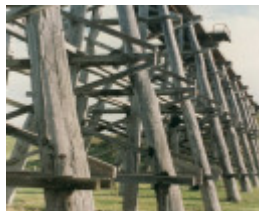
B7086 Nimons Bridge piers
