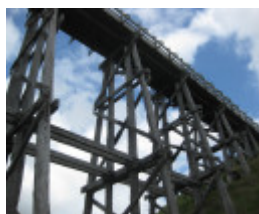
B7086 Nimons Bridge 2011
