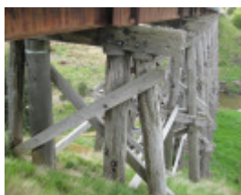
B7086 Nimons Bridge
