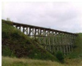
B7086 Nimons Bridge 2000
