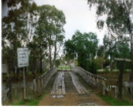
B6776 Condidorios Bridge
