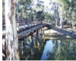
B6776 Condidorios Bridge
