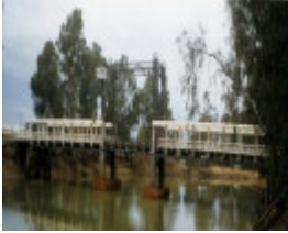
B4916 Barham-Koondrook Lift Bridge
