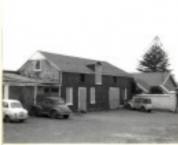
B0865 House Portland
