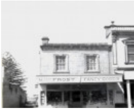
B0877 Shop upper storey before alterations
