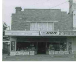
B0877 37 Julia Street - Upper Portion re-built
