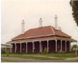
B2323 Lighthouse Keeper's Cottage Portland
