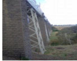
B5142 Moorabool viaduct
