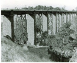
B5142 Moorabool Viaduct
