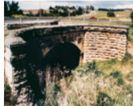
B2643 Waurn Ponds Bridge
