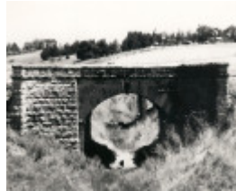
B2643 Waurn Ponds Bridge
