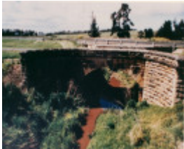
B2643 Waurn Ponds Bridge
