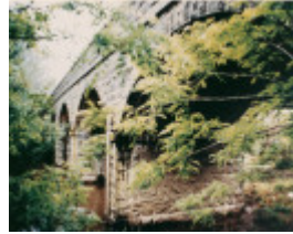
B1339 Bluestone Bridge Ballarat Rd Batesford
