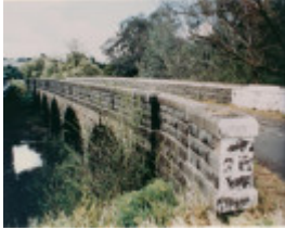
B1339 Bluestone Bridge Ballarat Rd Batesford
