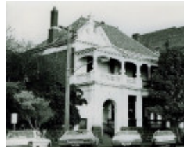
B3771 Fmr Corio Terrace
