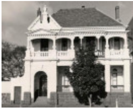
B3771 Fmr Corio Terrace
