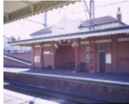
1 malvern railway station complex station street malvern south elevation apr1997
