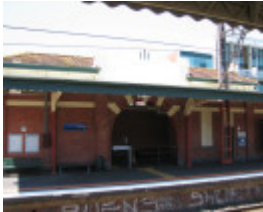
MALVERN RAILWAY STATION SOHE 2008
