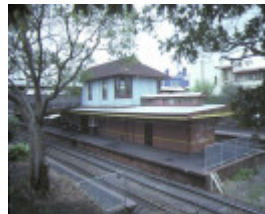
malvern railway station complex station street malvern end view sep1984
