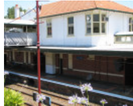
MALVERN RAILWAY STATION SOHE 2008
