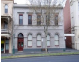
B3980 Fmr Bank of NSW
