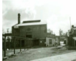
B5278 Bendigo Gasworks
