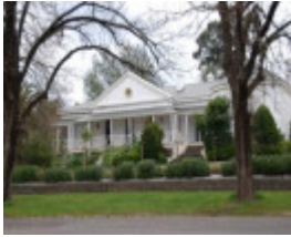
B0047 Bungalow - Former Post Office
